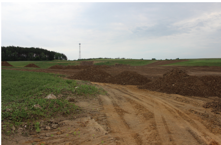
Fig. 2. Technical reclamation – prisms of humus earth used for reclamation in the Kanigowo VII mine
