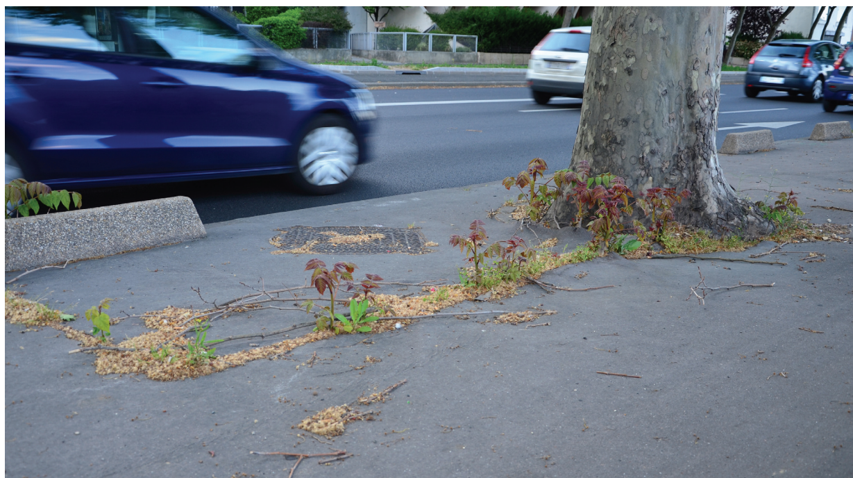
Fig. 5. Cracked, discontinuous surface of Ekranosol destroyed by plant roots (photo C. Kabała)
